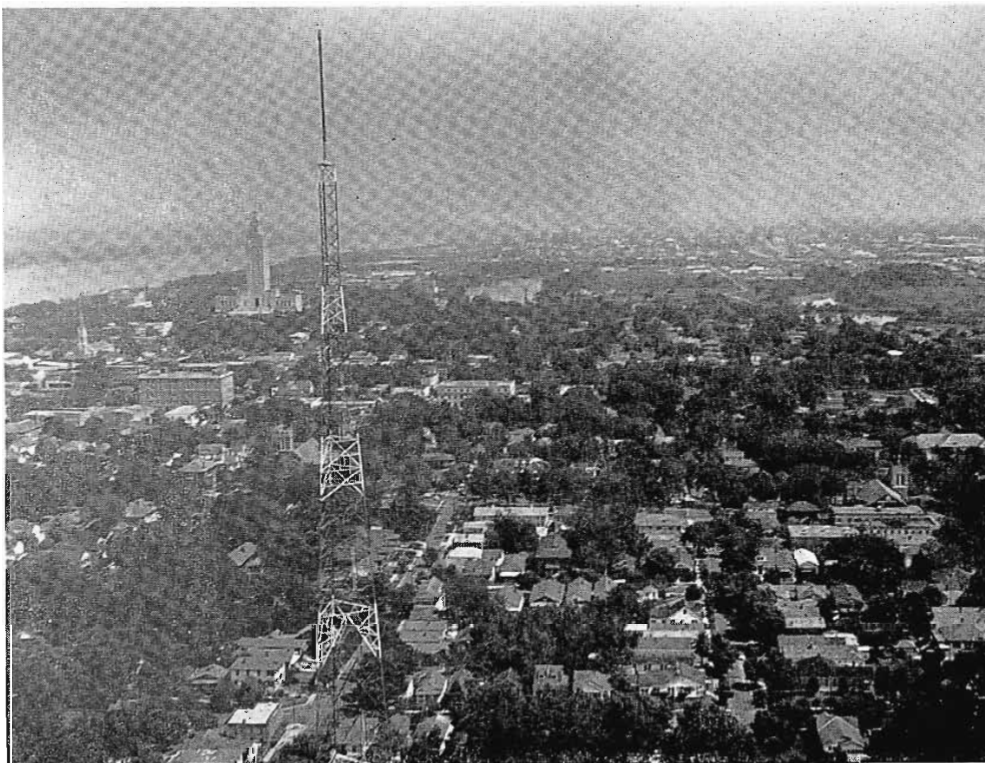
Below: WAFB-TV's tower and RCA 21-BL antenna rises 501 feet above the ground. The fabulous State Building—the house that Huey (Long) built—appears in the upper left portion of the picture.
